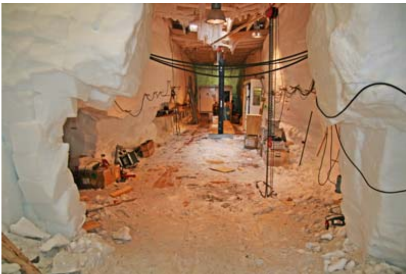
The drill trench without the winch and tower
