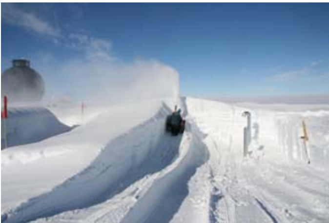
Removing snow from Drill Trench Roof
