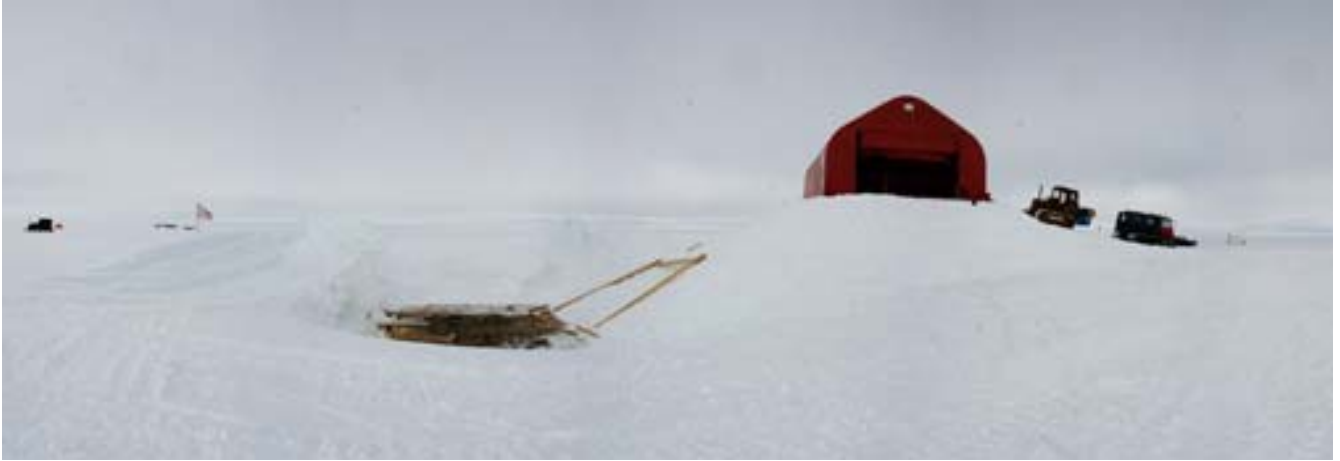
Garage move: The carpenter garage has been move to a new hill. The previous site was in the hole to the left. That hole was a 2 m hill in 2008 and illustrates the amount of snow accumulated in NEEM camp. For size comparison, note the Caterpillar tractor to the right of the garage.
