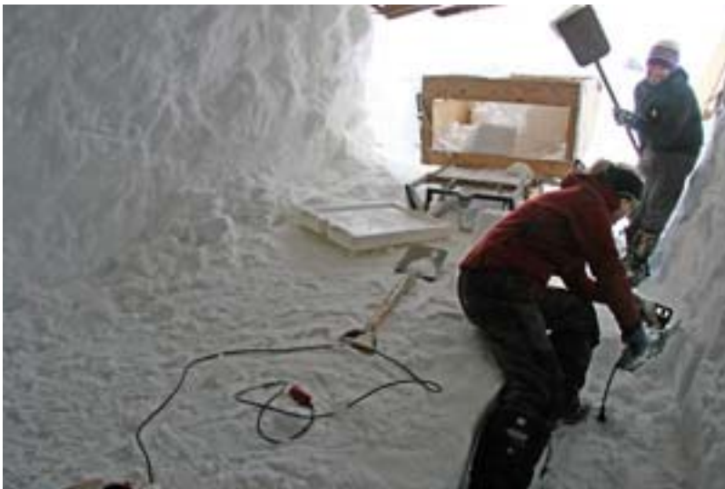
Helle and Paul busy with the chain saw lowering the floor in the drilling trench ramp.
