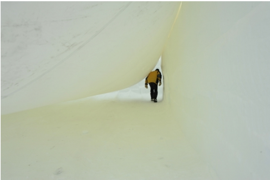
Inspection: A view from underneath the gas tank shows the size of the tank. J.P. inspects the position of the tank.
