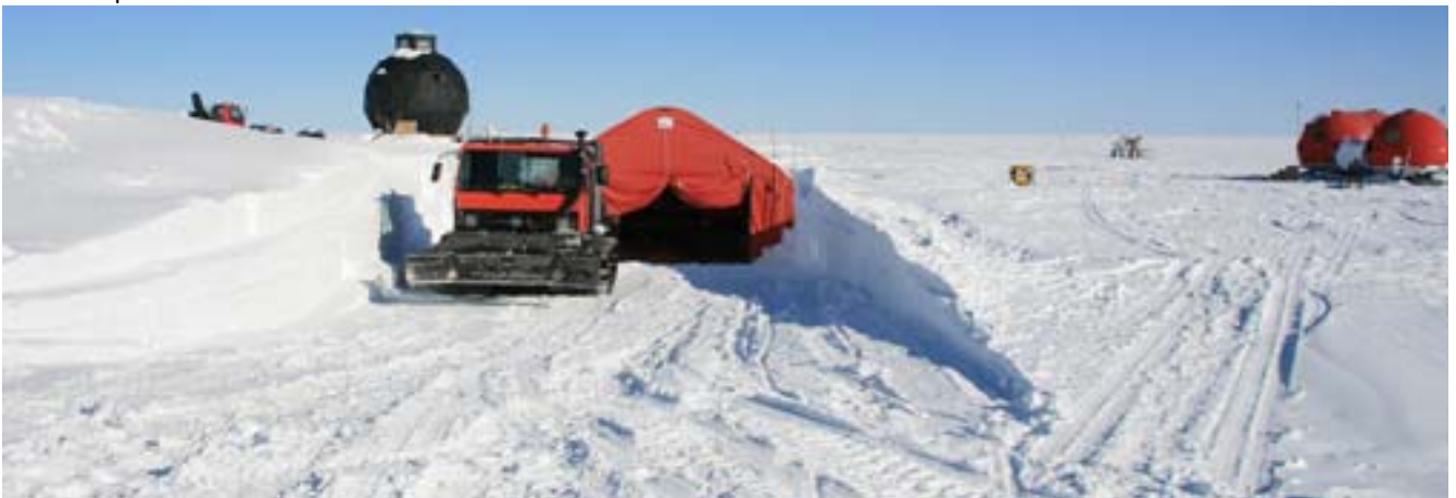
Mech garage: The newly excavated access ramp to the mechanics garage.
